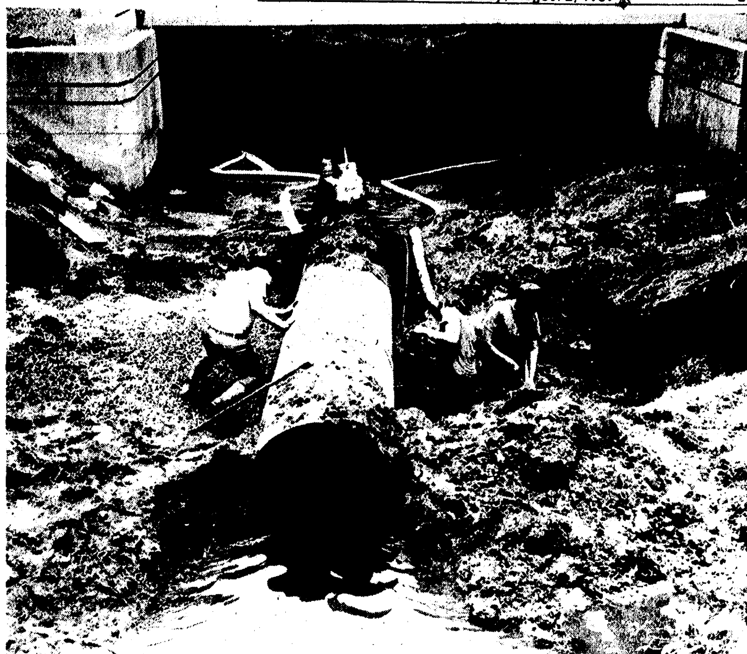
A SEWER FORCE MAIN had to run under Letts Creek on the north end of the village, and this is how workers managed to get the water out of the way to install the pipe. The pipe carried the water while workers concentrated their efforts underneath. Pumps got rid of any water that seeped into the work area.
